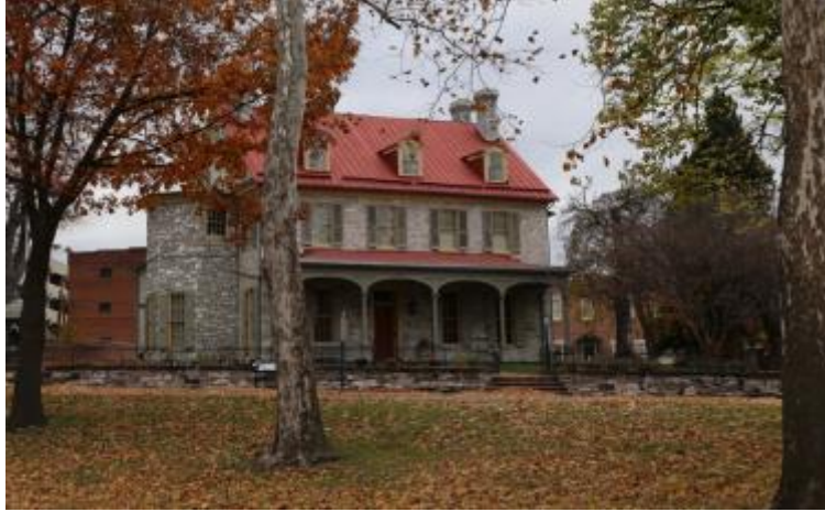
This is the Harris/Cameron Mansion in Harrisburg, PA.
